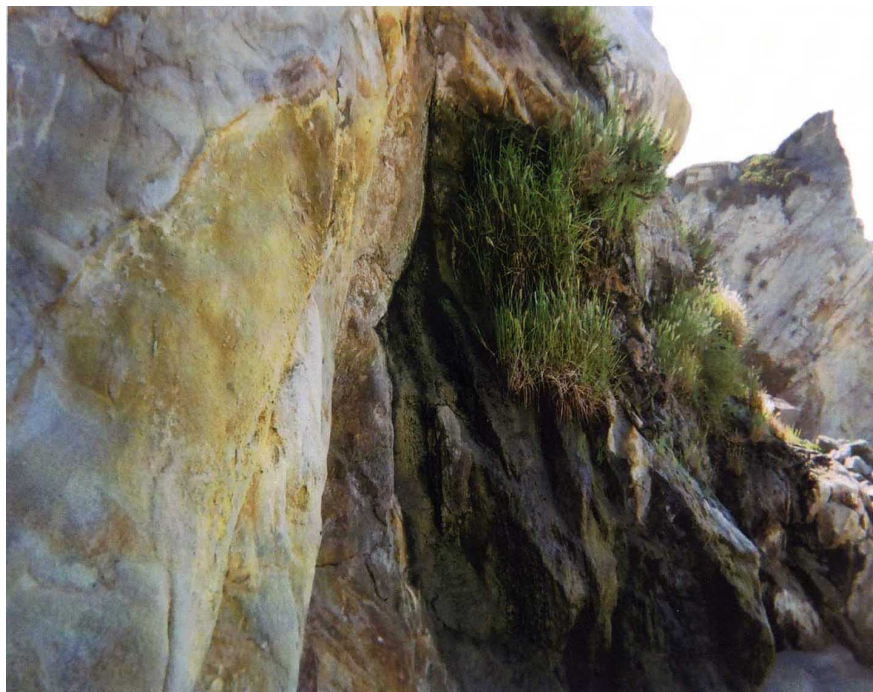
Figure -8 Second fault exposure that runs at a right angle from promontory fault. Note yellow sulfur stain precipitated from mineral spring.
