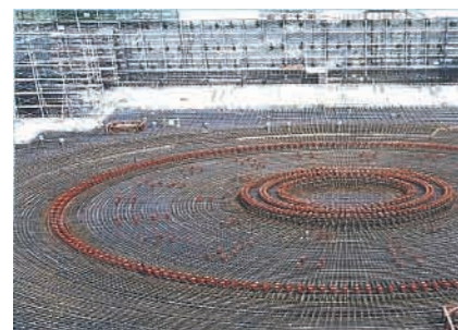
Rebar assembly of the base mat of the reactor building
