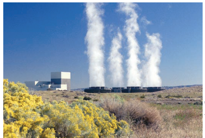
Columbia Generating Station in Washington topped this year's list with three incidents that led to special inspections.
