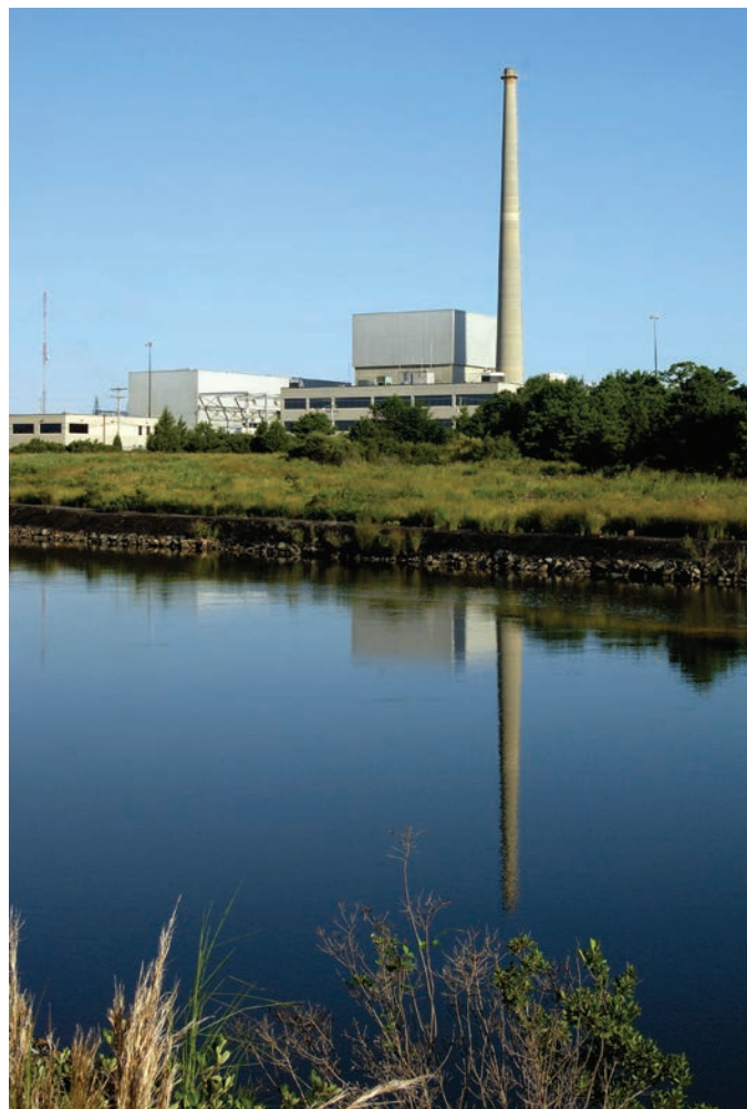
Oyster Creek nuclear plant in New Jersey lost offsite electrical power following Hurricane Sandy.
