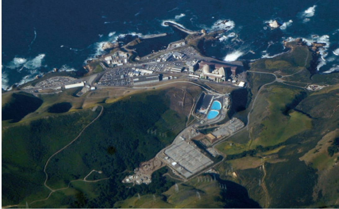
The NRC has not enforced seismic regulations at the Diablo Canyon plant in California as it has at other nuclear plants.
