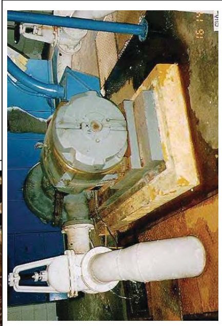
Figure 5-3: Large horizontal pumps like the DCPD heater drain pump (upper left) are present in many forms at sites investigated for the EPR database. Examples include circulating water pumps, such as the unit at the Valley Steam Plant at upper right, and feedwater pumps such as the units serving the Manzanillo Steam Plant at lower left. Variations on large feedwater pumps include steam-turbine-powered units, such as at the Pasadena Power plant at lower center. Serious earthquake damage to horizontal pumps is rare. One of the few instances occurred in the Island of Guam water system, where motors required replacement on two pumps (lower right) due to apparent pressure surges in the downstream pipelines.
