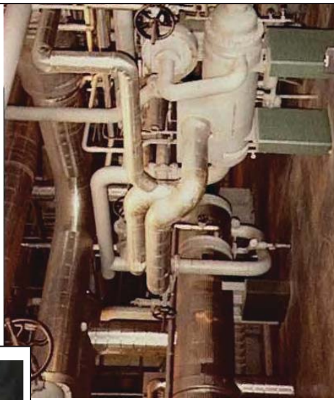
Figure 5-7: Essentially all steam generating units include one item of steam-plant-specific equipment. An example is the lube oil tank and pumps for the DCCP at upper left. The lube oil tank at one of the Burbank steam units is shown at upper right. The main steam condenser and the gland steam condenser for one of the units at El Centro are shown at lower left and lower center. At lower right is the lube oil conditioner for one of the steam units at Humboldt Bay. Within the data sample of some 20 of the larger steam generating units operating at the time of their earthquake, there are no instances of serious damage to steam-plant-specific equipment.
