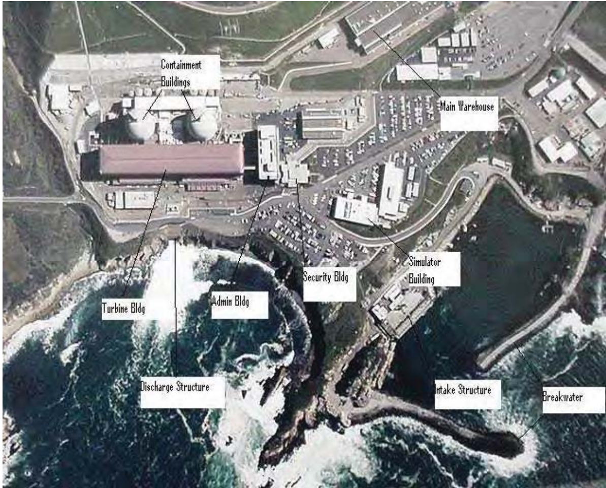
Aerial View of Power Block Showing Various Buildings
