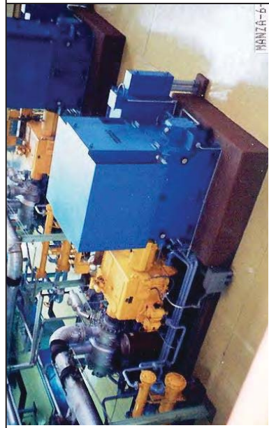
Figure 5-3: Large horizontal pumps like the DCPD heater drain pump (upper left) are present in many forms at sites investigated for the EPR database. Examples include circulating water pumps, such as the unit at the Valley Steam Plant at upper right, and feedwater pumps such as the units serving the Manzanillo Steam Plant at lower left. Variations on large feedwater pumps include steam-turbine-powered units, such as at the Pasadena Power plant at lower center. Serious earthquake damage to horizontal pumps is rare. One of the few instances occurred in the Island of Guam water system, where motors required replacement on two pumps (lower right) due to apparent pressure surges in the downstream pipelines.
